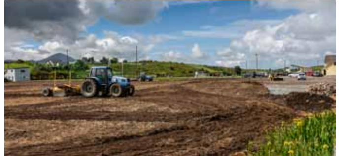
Pitch under construction
